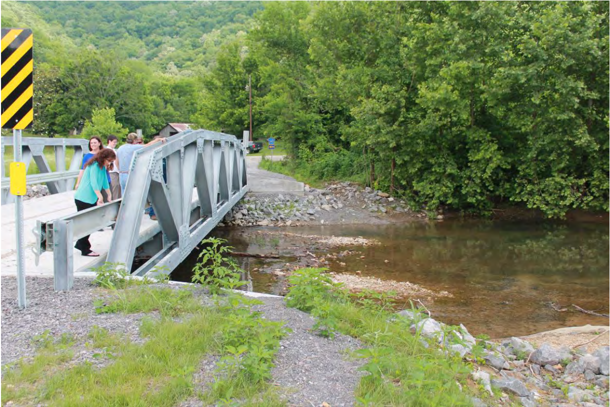
Replacement of low water crossing/fish barrier by bridge, Estill Fork.
