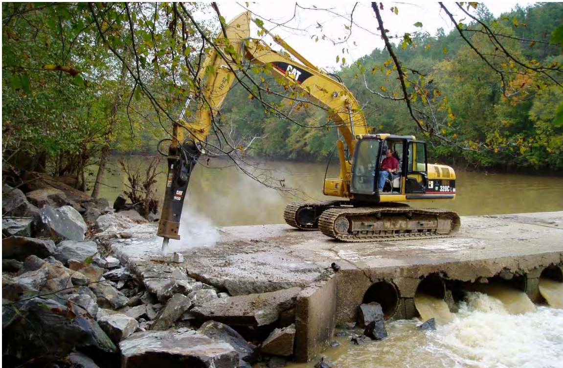
Figure 3-17. Removal of the Marvel Slab dam on the Cahaba River, 2004
