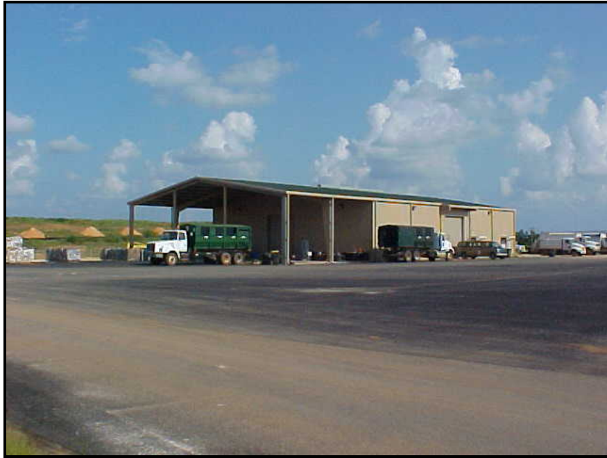
Household Hazardous Waste Handling and Disposal Facility /Recycling Center located at Magnolia Landfill in Summerdale, AL. The facility was constructed in 2006 with funds from the previous CIAP.
