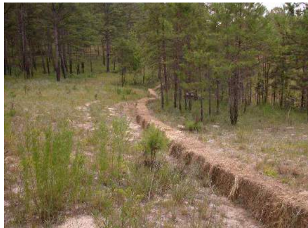
View of completed hay bale pen along south side of enclosure looking east.
