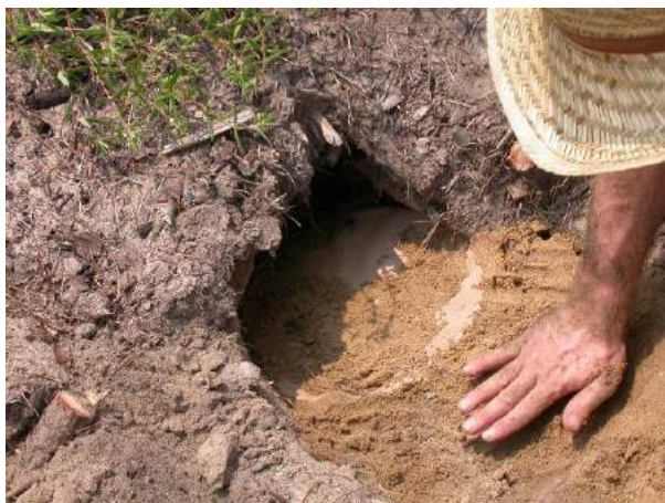
Sand is packed against packaging paper to keep it tight over the bucket.
