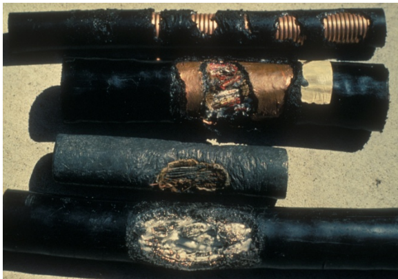
Figure 8. Utility cables gnawed by pocket gophers. Photo by UNL.
