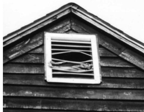
Figure 6. A raccoon entered this attic through the vent. Photo by Stephen M. Vantassel.
