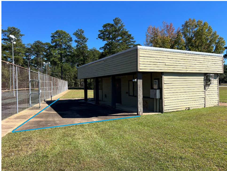
RESTROOM NORTHWEST CORNER
