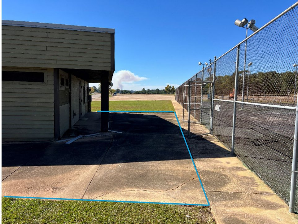
RESTROOM NORTHEAST CORNER
