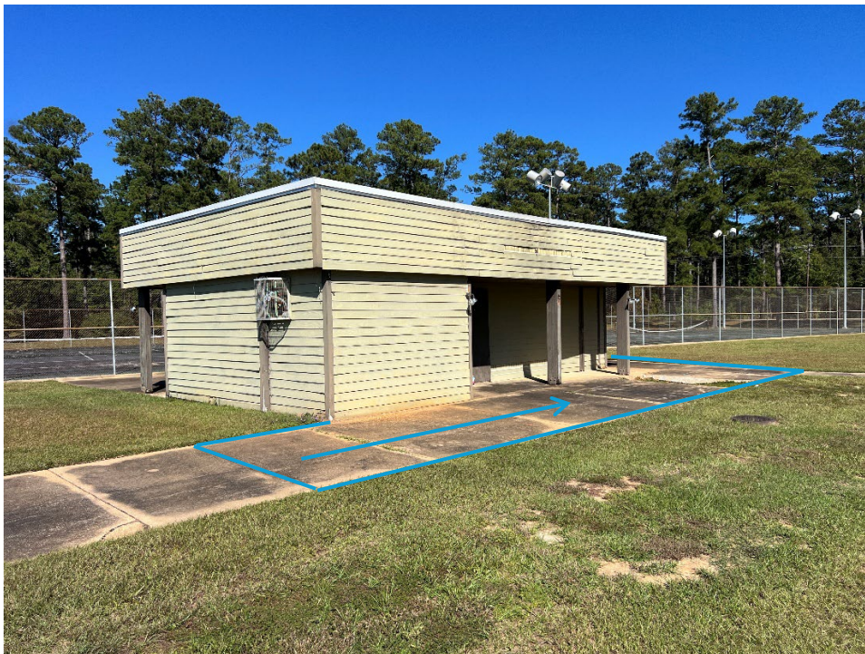
RESTROOM SOUTHWEST CORNER
