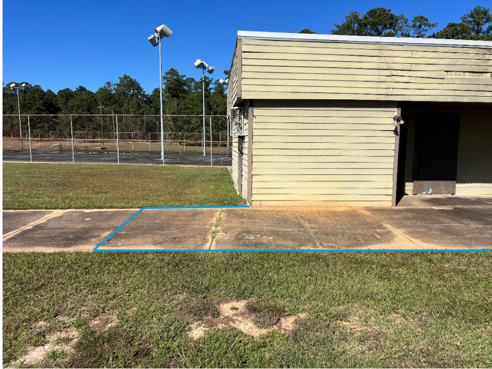
RESTROOM SOUTHWEST CORNER LOOKING NORTH
