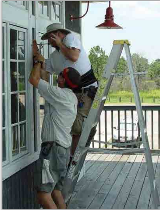
Installing hurricane protection
