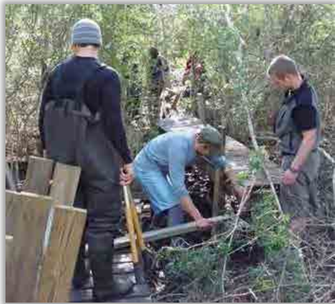
AmeriCorps volunteers repair research boardwalk
