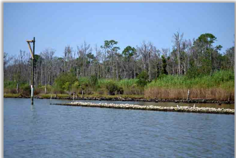
A living shoreline protects and helps restore eroded bayfront along Bon Secour Bay
