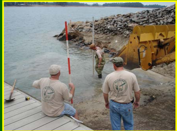
S.B. Pope measures the depth prior to a ramp extension while Mike Hale (left) and Steve Taylor (right) prepare to add gravel to achieve the proper slope of 15 %.
