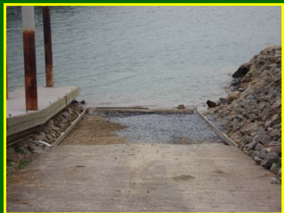
The resulting void is ready to be reinforced with rebar and filled with fresh concrete.
