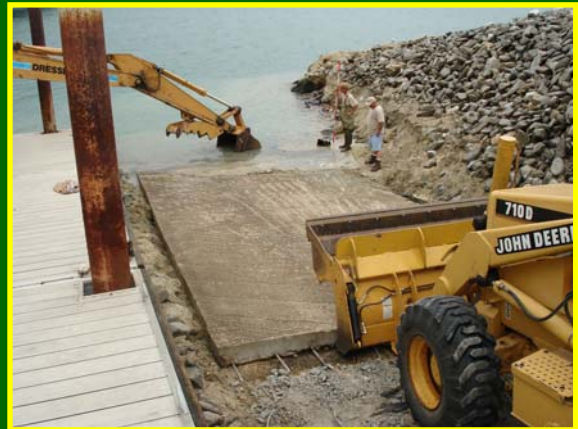
The last 30 feet of an existing boat ramp is cut off and carefully pushed into place by Tim Brewer (backhoe operator).
