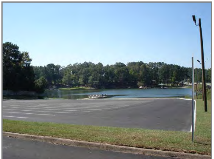
At Lake Eufaula, parking was expanded at the public ramp at Thomas Mill Creek. This project was completed in cooperation with the Henry County Commission.
