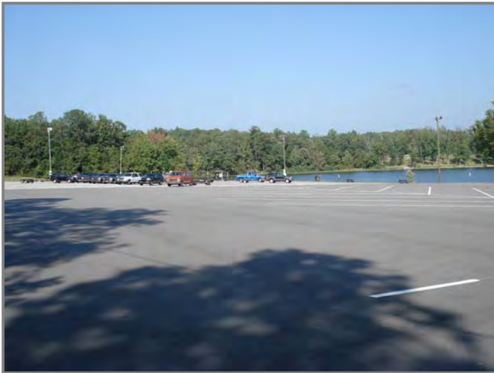
The parking area at Beeswax Creek on Lay Lake was expanded to include parking for more than 70 trailers and striping plans were engineered to improve traffic flow and accommodate larger rigs. This project was completed in cooperation with Alabama Power Company.
