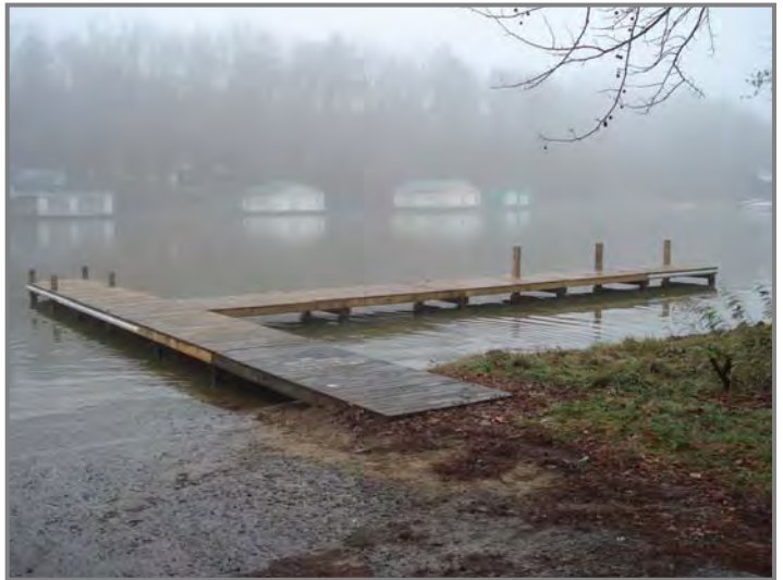
At Lake Guntersville, an new wharf-style pier was added at Waterfront to replace an aging courtesy pier. This site is also scheduled for a ramp replacement during February, 2009.
