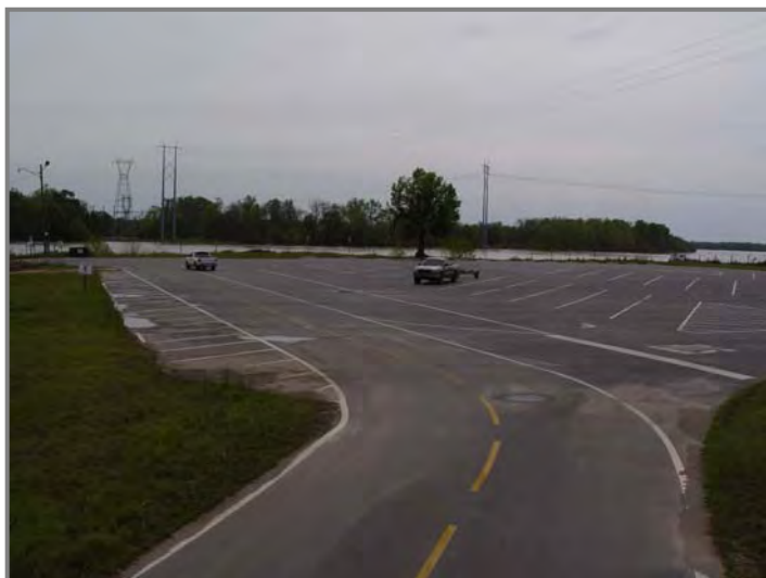
In the Mobile Delta, parking was expanded to make room for 36 rigs at the Mt. Vernon Boat Ramp. A gravel overflow parking area will be added during summer 2009.
