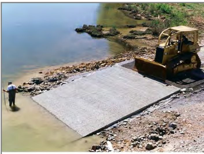
At Claiborne Landing off Hwy. 84 in Monroe Co., a new boat ramp was constructed to replace an old, inadequate ramp.
