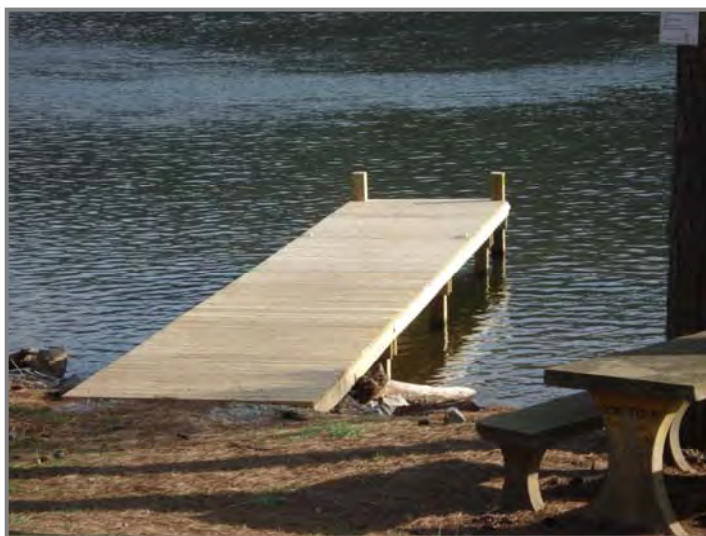
On Lake Guntersville, a new courtesy pier was constructed at Town Creek Boat Ramp.
