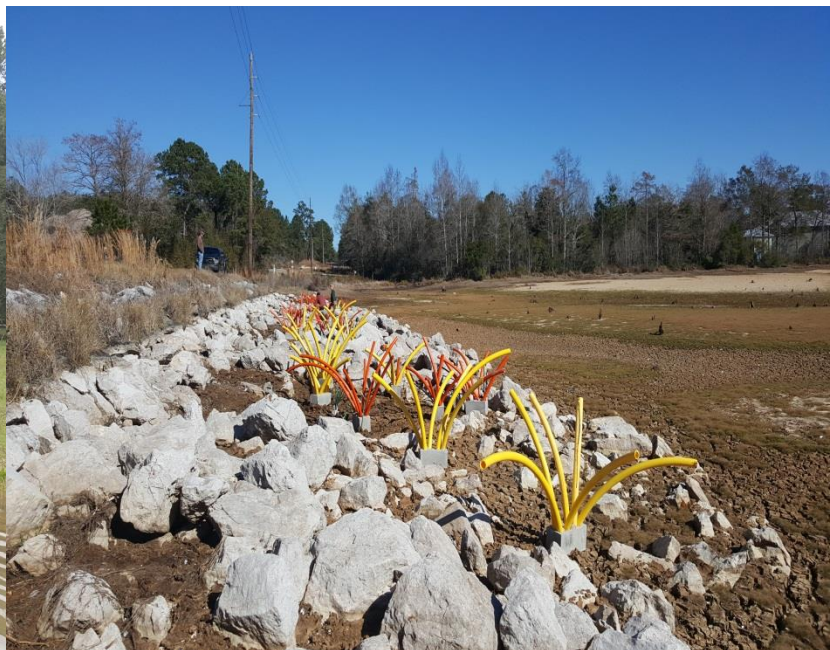
Spiderblocks installed during Point A Reservoir drawdown
